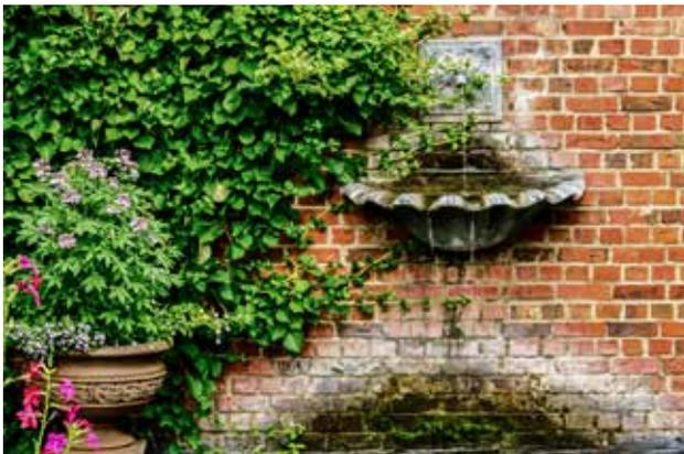
Most of these deposits were once water-soluble salts that could have come from many possible sources and have been deposited on the substrate surface as the water that carried them has evaporated naturally.
